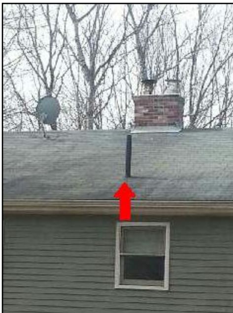
3. Top of flashing exposed or bottom buried
